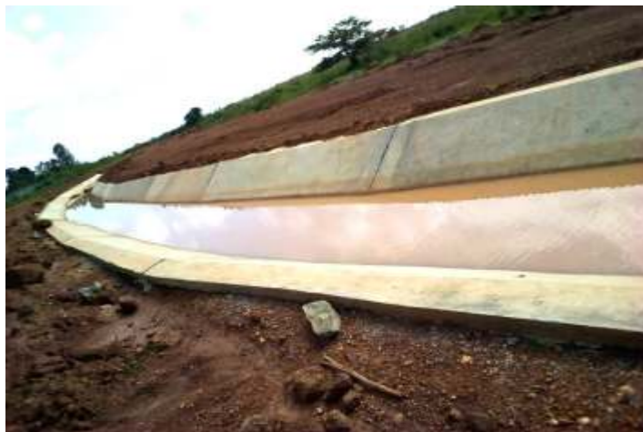
A primary canal filled by rain water at Tochi Irrigation scheme
