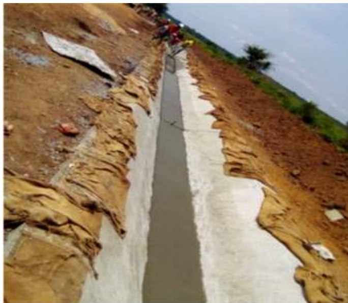
Secondary canal under construction at Wadelai Irrigation Scheme
