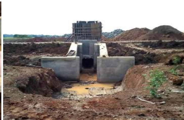
The Left-hand regulator at Tochi Irrigation scheme
