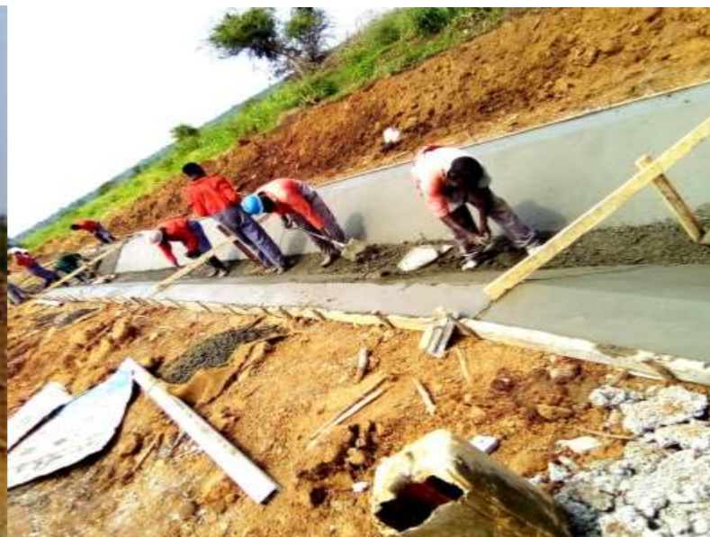
Secondary canal under construction at Wadelai Irrigation Scheme
